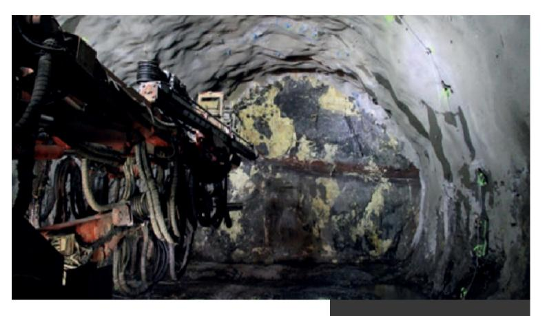
The injection sealing made use of Carbopur WX and accelerators, while at extreme cases at the location, Carbopur WF and additives were injected.
