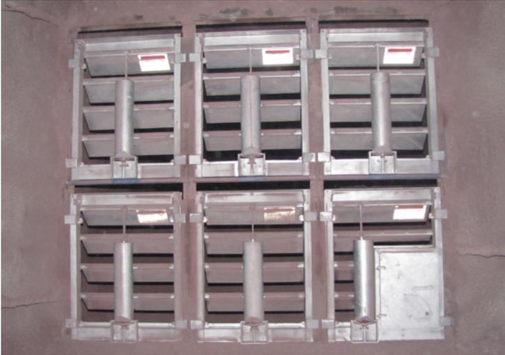
**Blastflow louvre regulators provide enhanced control of airflow in primary ventilation circuits which are subject to air overpressures from stope firings.**
