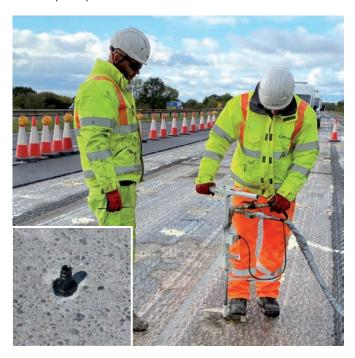
The process is continuously monitored using geodetic equipment. Packer surfaces are mechanically removed and any excess resin is removed from the road surface.
