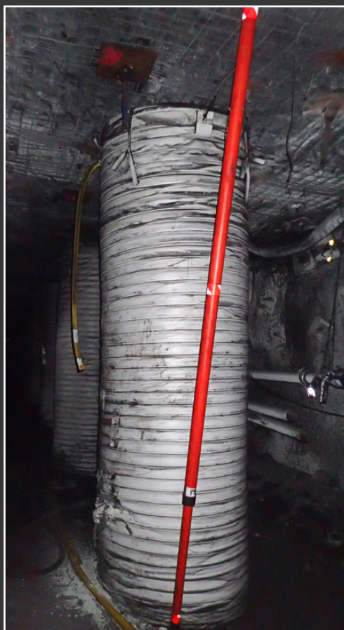
Installed pumpable crib
